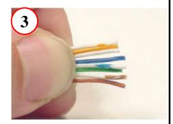
**Position Wires into Correct Configuration (586-B Shown)**
